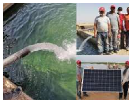
147KW solar water pump system in Saudi Arabia
