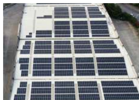
Hsu Fu Chi International Co., Ltd. Installed Capacity: 5170kWp
