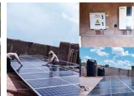
30KW off-grid solar system in DRC
