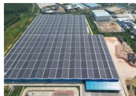
Shuncheng Ceramic Group Installed Capacity: 5112.7kWp
